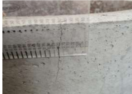
Figure 11 (b): Photo showing crack and crack width measurement
