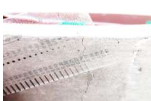
Figure 10 (b): Photo showing crack and crack width measurement
