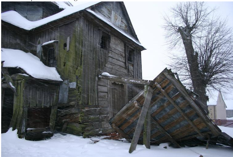
Fig. 3. Greek-Catholic church in Miękiszy Stary – collapsed porch adjacent to the women's porch from the west; photo T. Tomaszek.
