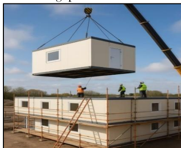
Fig. 1 On-site Construction of Modular Building
