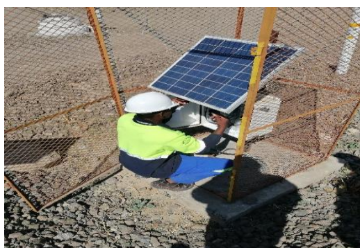
Fig. 7: A Piezometer Station
