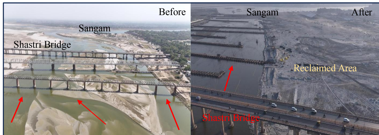
Fig. 8 Drone view of before and after dredging of Ganga River from upstream shastri bridge
