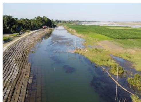
(Photo Plate 6)- The embankment work under the recently funded World Bank project in the Bardanga Khatakuchi region has been instrumental in reducing the erosion of the Beki River, demonstrating the effectiveness of targeted interventions in
