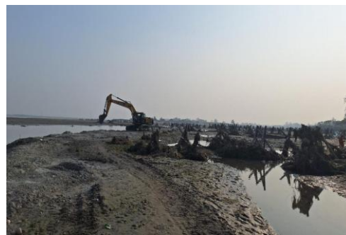
(Photo Plate 2)- Recent embankment work, including the placement of porcupines, is seen nearby Beki Bridge to reduce the current of the Beki River over NH-31.
