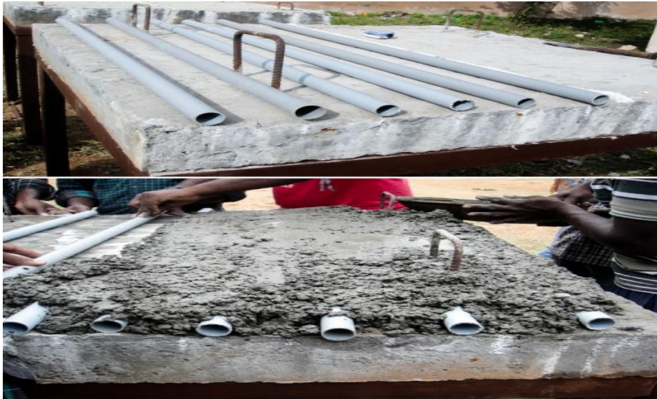
Fig 4 RC slab with air transient layer
