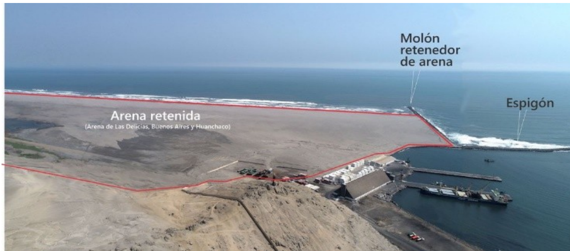
Figure 5. Coastal sediment retained by the breakwater jetty at the Port of Salaverry.
