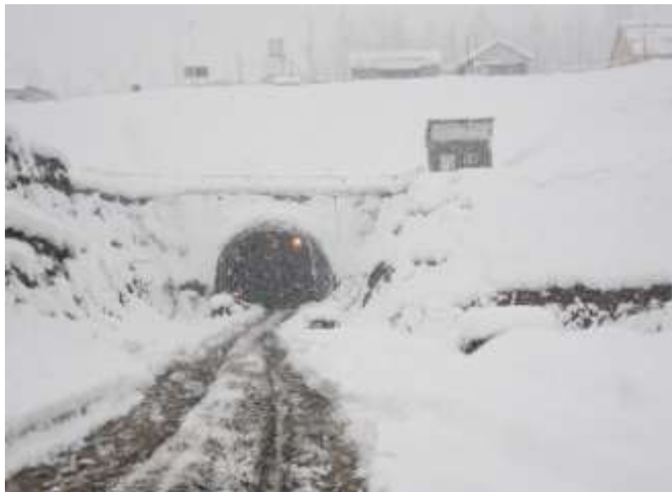
Fig: 1 Source: https://www.cecr.in/underground-construction-1/conventional-tunnelling-challenges-in-the-himalayas-a-case-study
