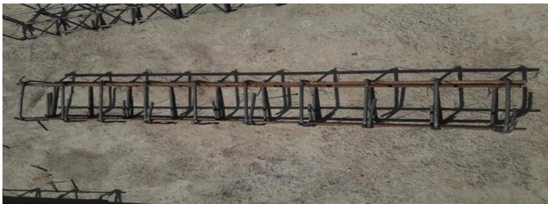
Fig 7 Reinforcement of Beam
