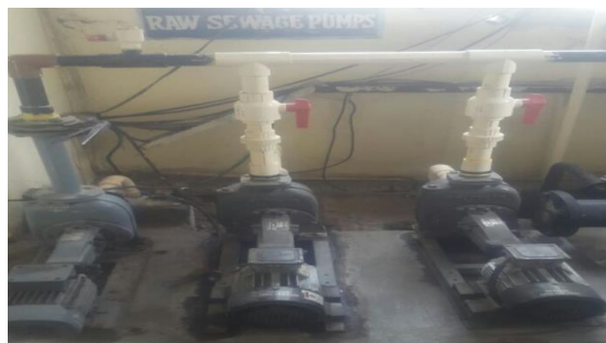
Fig.3 Raw Sewage Treatment Pump
