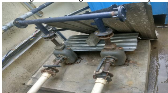
Fig.5: Return Sludge Pump
