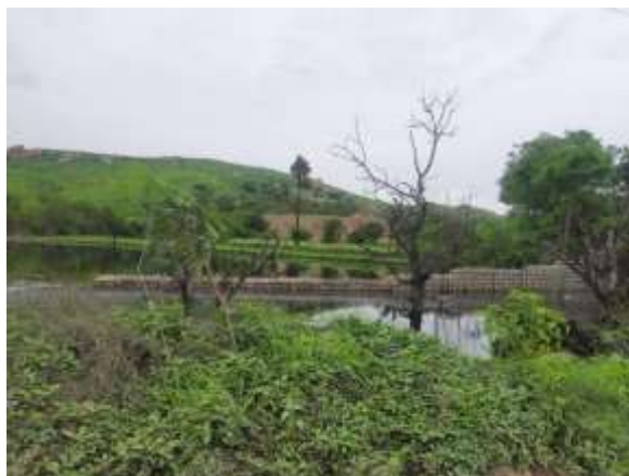
Figure 3: Landscape view of Jawahar Nagar landfill showing leachate stagnation and uncapped waste zones
