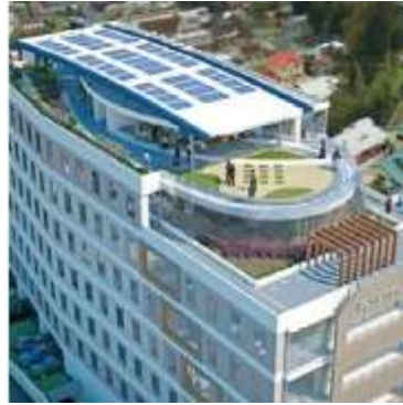
Fig. 1 Savannah East Building Trinidad and Tobago [7]
