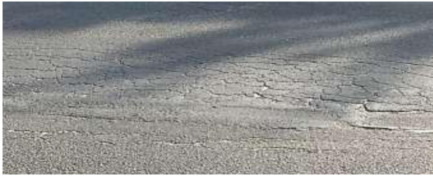
Figure 3. Alligator crack on distressed section
