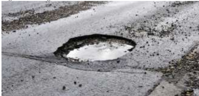
Figure 4. Pot holes on the highway section under study
