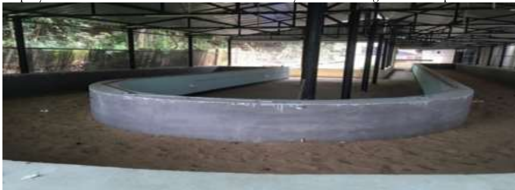
Figure 1. 180° bend in the channel
