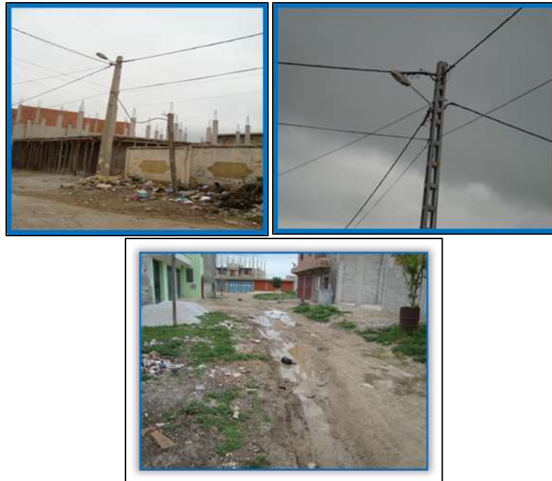
Figure 10: observed infrastructure deficits in the study area (authors)
