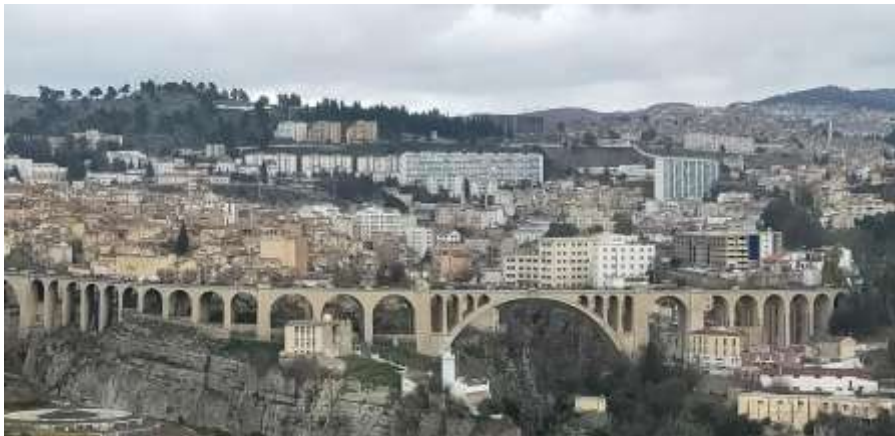
Figure 5. Sidi Rached Bridge ( Note: By Nadira Bouguebs, 2025 )
