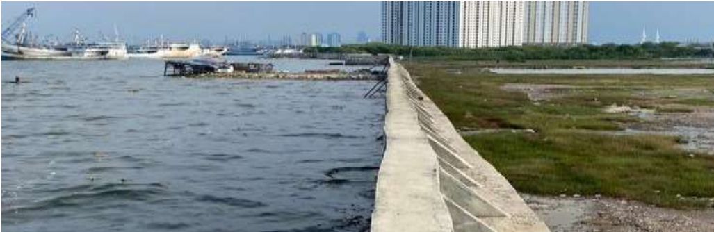
Figure 5. Coastal Erosion Control Embankment
