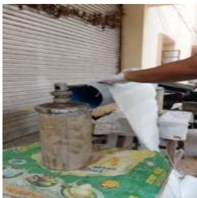
Figure 2 Application of GFRP sheet
