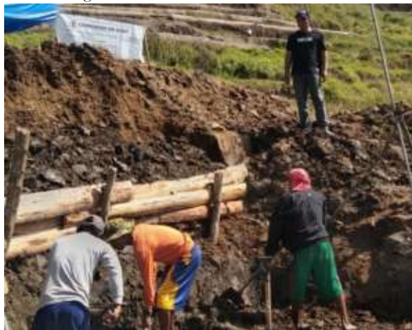
Figure 7. Placement of wooden logs to avoid further erosion of the debris
