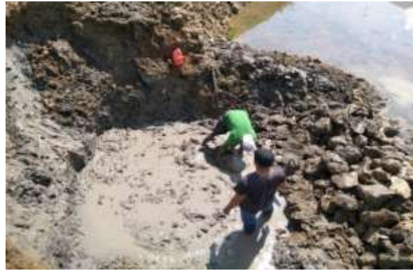
Figure 8. Excavation and dewatering process in the wall foundation preparation
