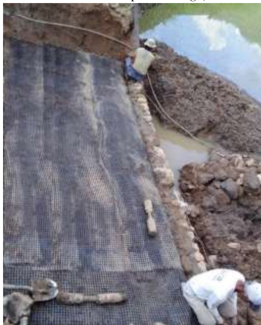
Figure 9. Geogrid placement in compacted layers
