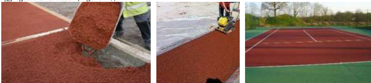
Figure 17. The use of permeable flooring: porous concrete. Source: author's archive.
